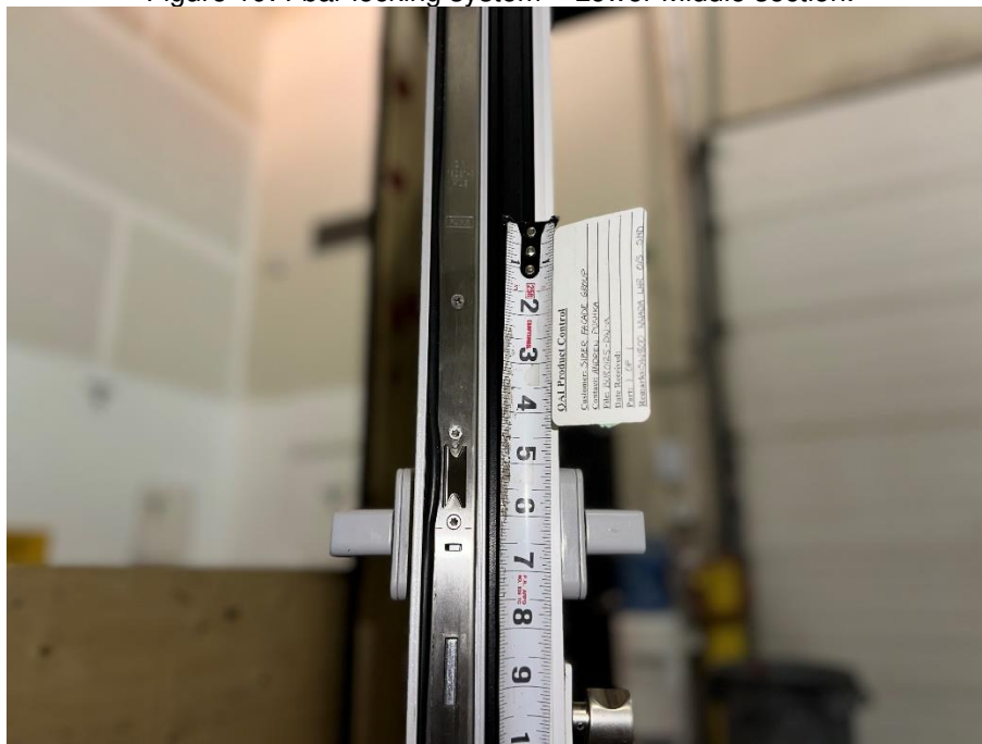
Figure 20: I-bar locking system – Upper middle section.
