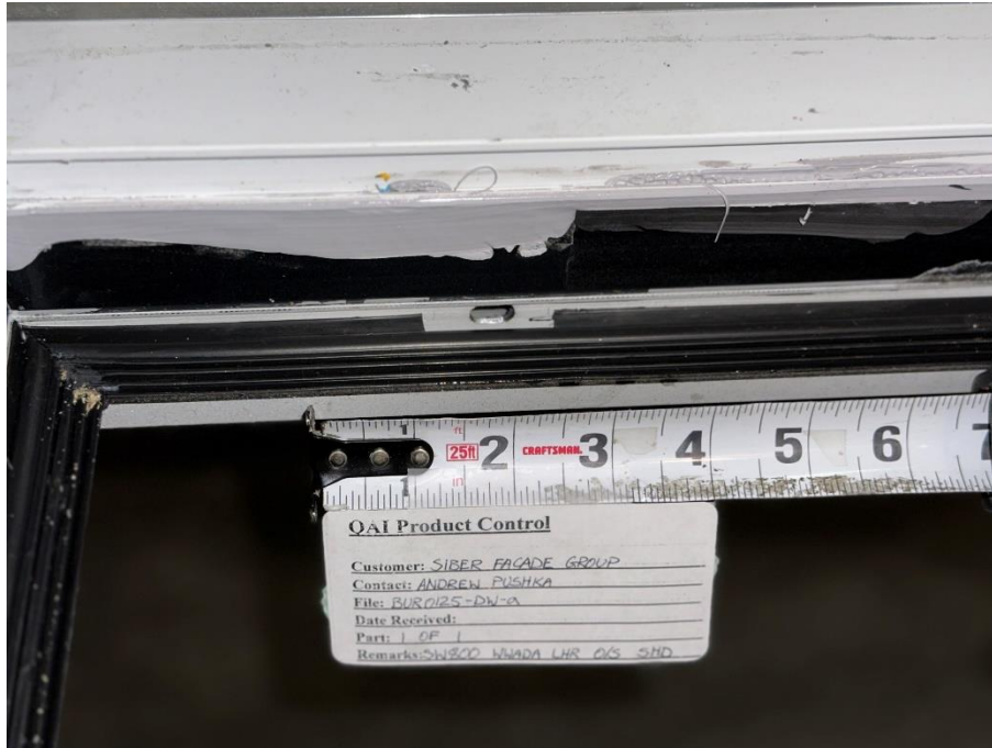
Figure 15: Drainage into the door slab.
