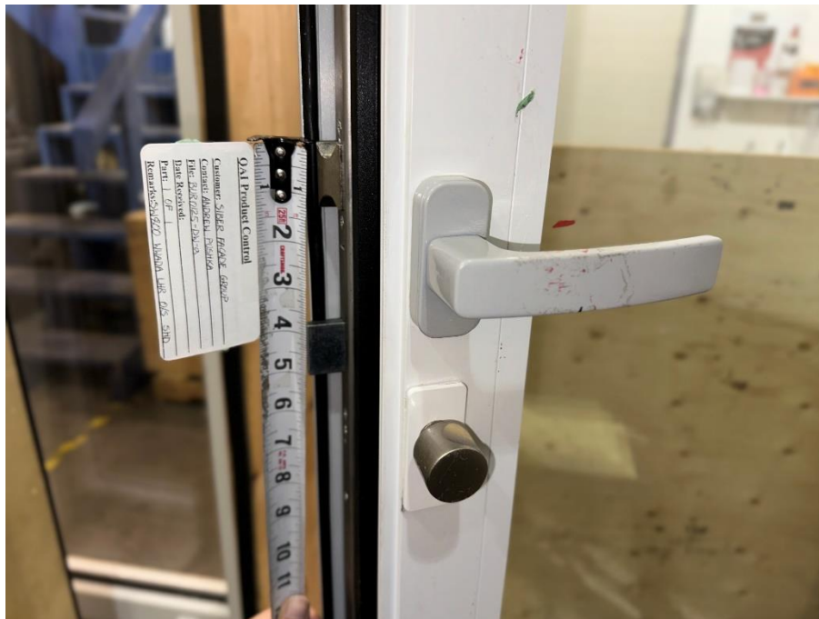
Figure 26: Lever handle and thumb turn operators.
