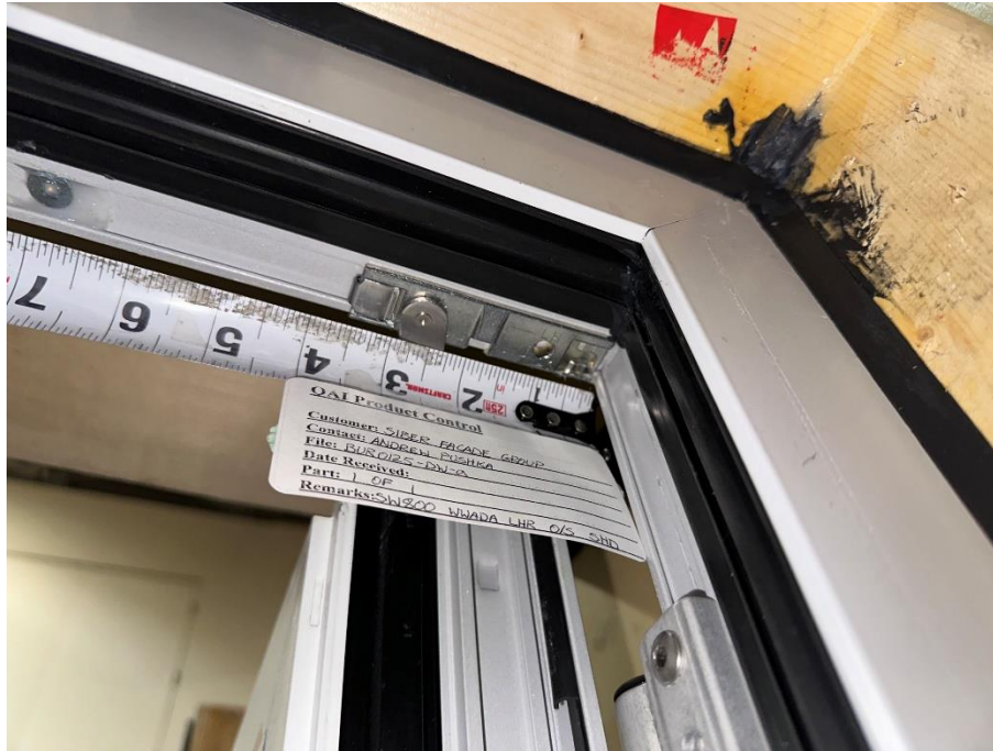
Figure 29: Stay arm hinge – Frame side.
