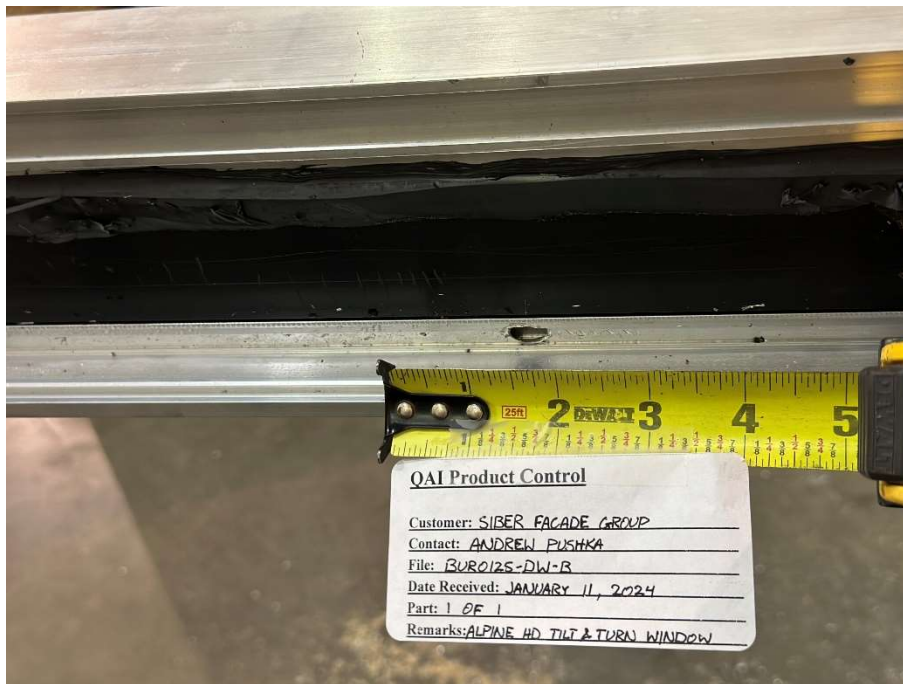
Figure 15: Drainage into the sash.
