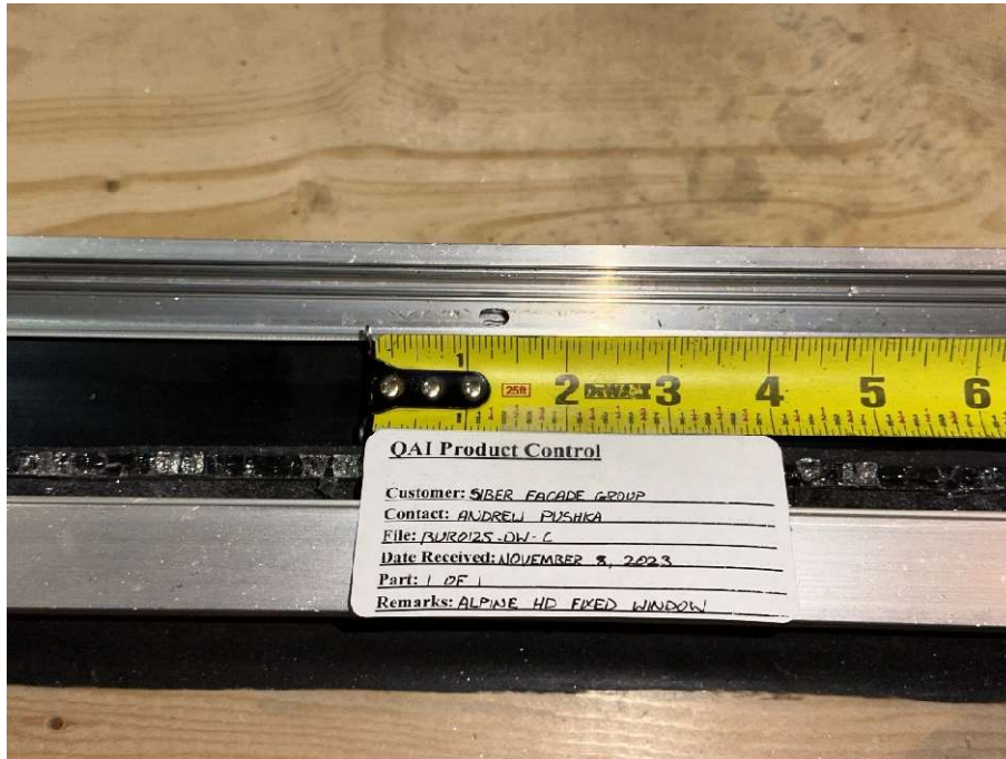
Figure 5: Drainage into the frame.
